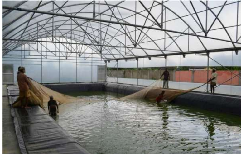
Photo-II: Concrete pond (320sqm) inside the polyhouse lined with black polyethene to prevent leakage, to enhance and retain water temperature.
