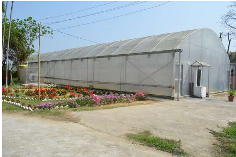
Photo-I: The polyhouse (420sqm) with filtration and heating systems constructed for artificial enhancement of environmental temperature for the study
